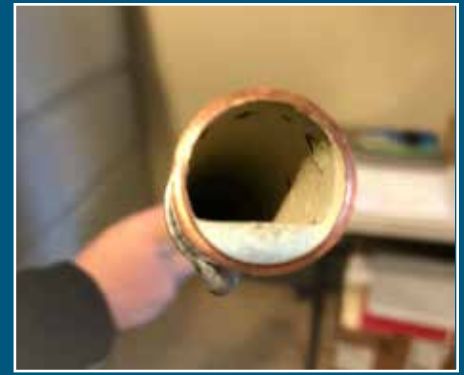
C. Pipe lining
